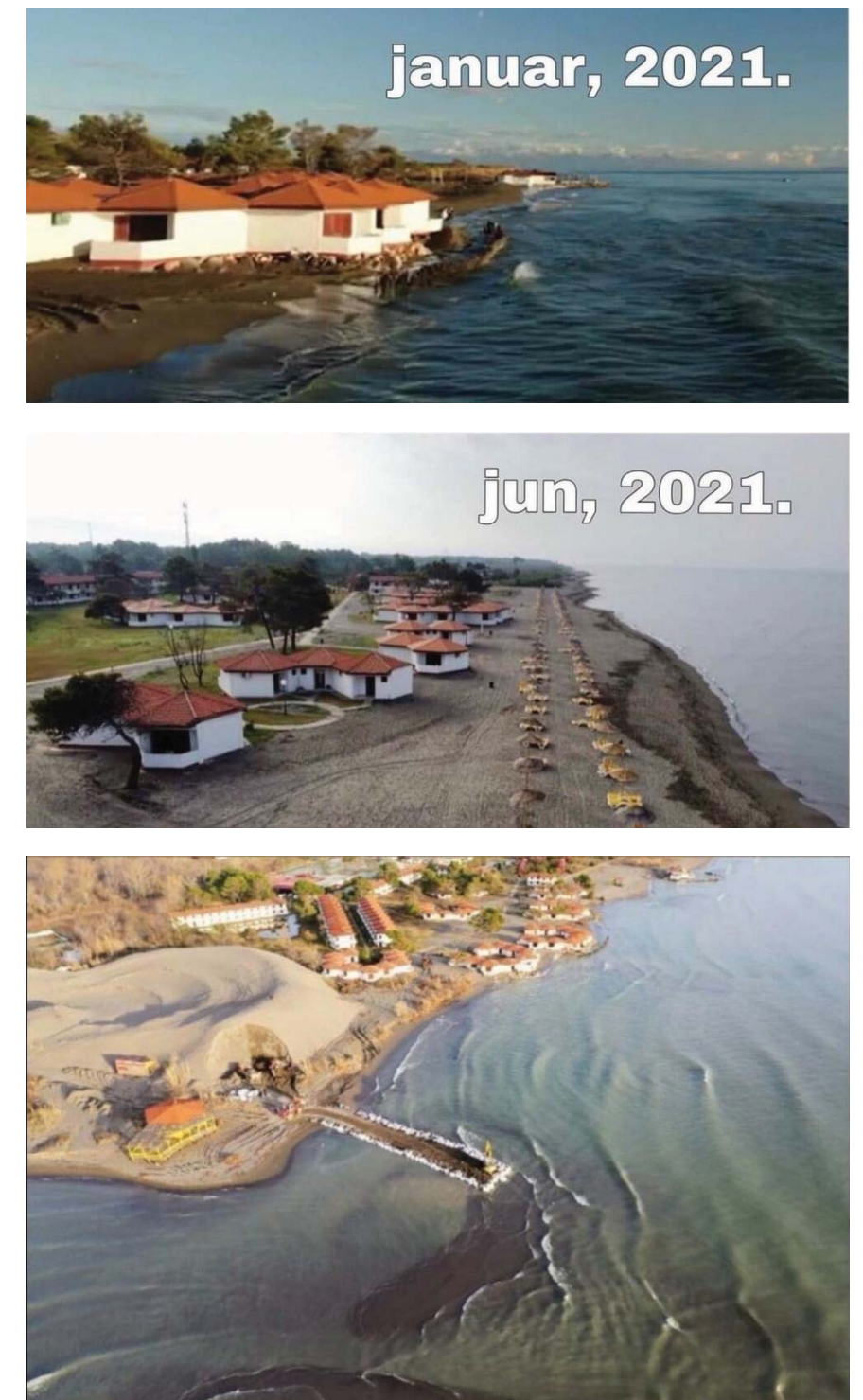
Figure 6.9. Urgent remediation measures (by placing sandy groyne and nourishing the beach with the sand from Bojana river dredging during previous years), temporarily stopped the erosion of the beach on the west side of Ada Bojana. Upper image- the situation in January 2021; middle image – June 2021 (PEMDM); bottom image – works in March 2021 (MESPU)..
