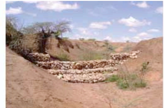
Plate 1 (left) depicts a badland while plate 2 (right) depicts a gully control measure (check dam implemented by IFAD)
