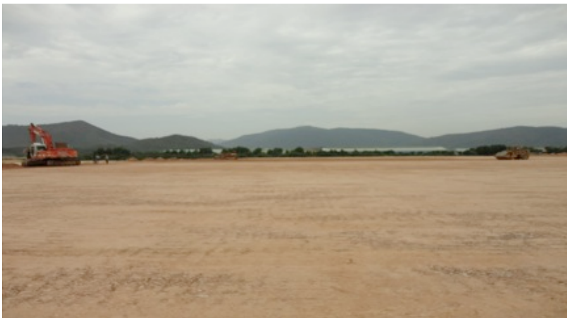
Site Filling Works for Ha Thanh WWTP using CEPT Technology - June 29, 2011
