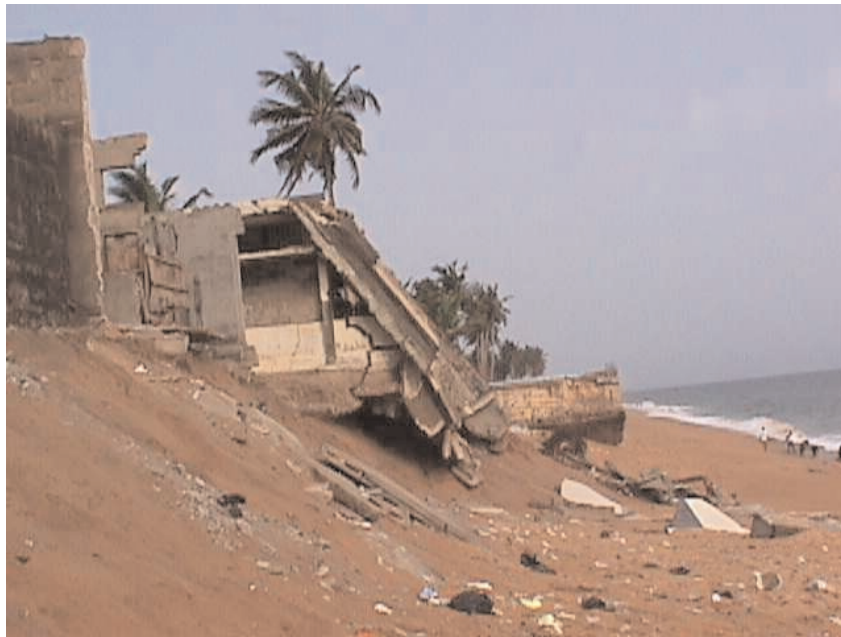
Photo 5.1: Typical example of acute coastal erosion (Port-Bouët, Côte d'Ivoire)
