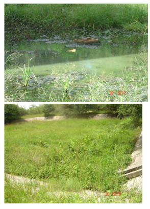
Images of over flowing sewage and sewage treatment pond over growing with weeds and shrubs at Max Makuse Secondary School.
