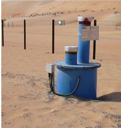
Well Head of Double Casing Monitoring Well in the ASR-Pilot Project Are
