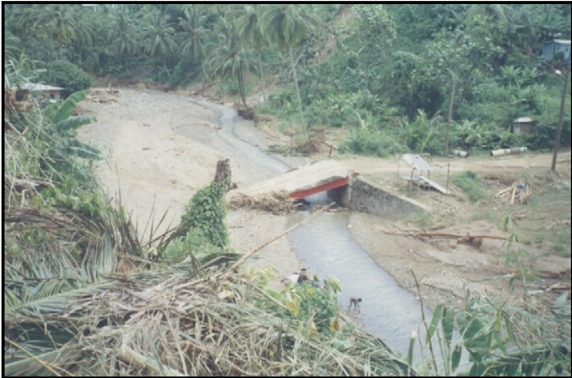
Fig. 2.6 : Destruction to Millet Bridge after Tropical Storm Debbie
