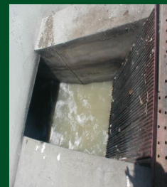
Preliminary treatment: bar screen.
