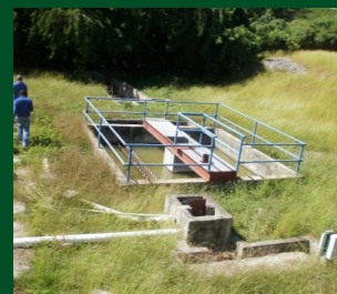
Clarifier, missing sludge pump and chlorination
