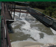
Secondary treatment: Aeration chamber
